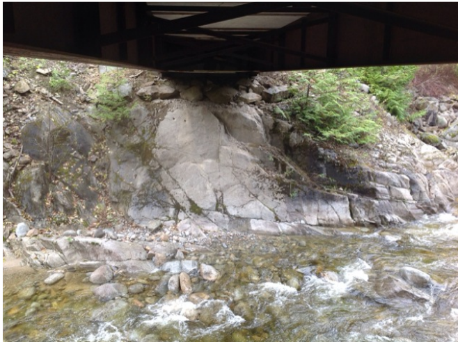
Right Bank Abutment when facing downstream
