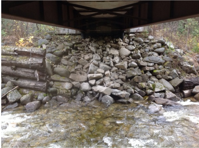
Left Bank Abutment when facing downstream
